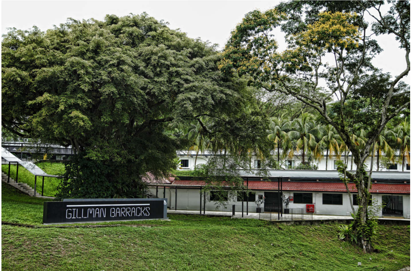
Figure 1. Gillman Barracks, Singapore.
